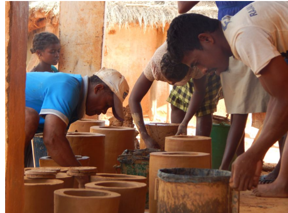
We work with local people to introduce sustainable income generating activities. Here, community members build energy efficient stoves.
